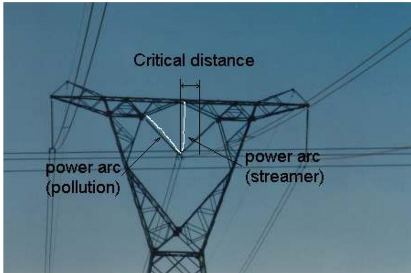
A distance of one meter either side of the conductor is regarded as critical in protection against streamer faults.
